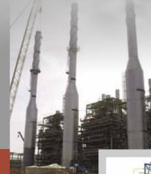
single drum type radiant boiler I fully-welded natural circulation I vertical gas path I bottom or top supported
